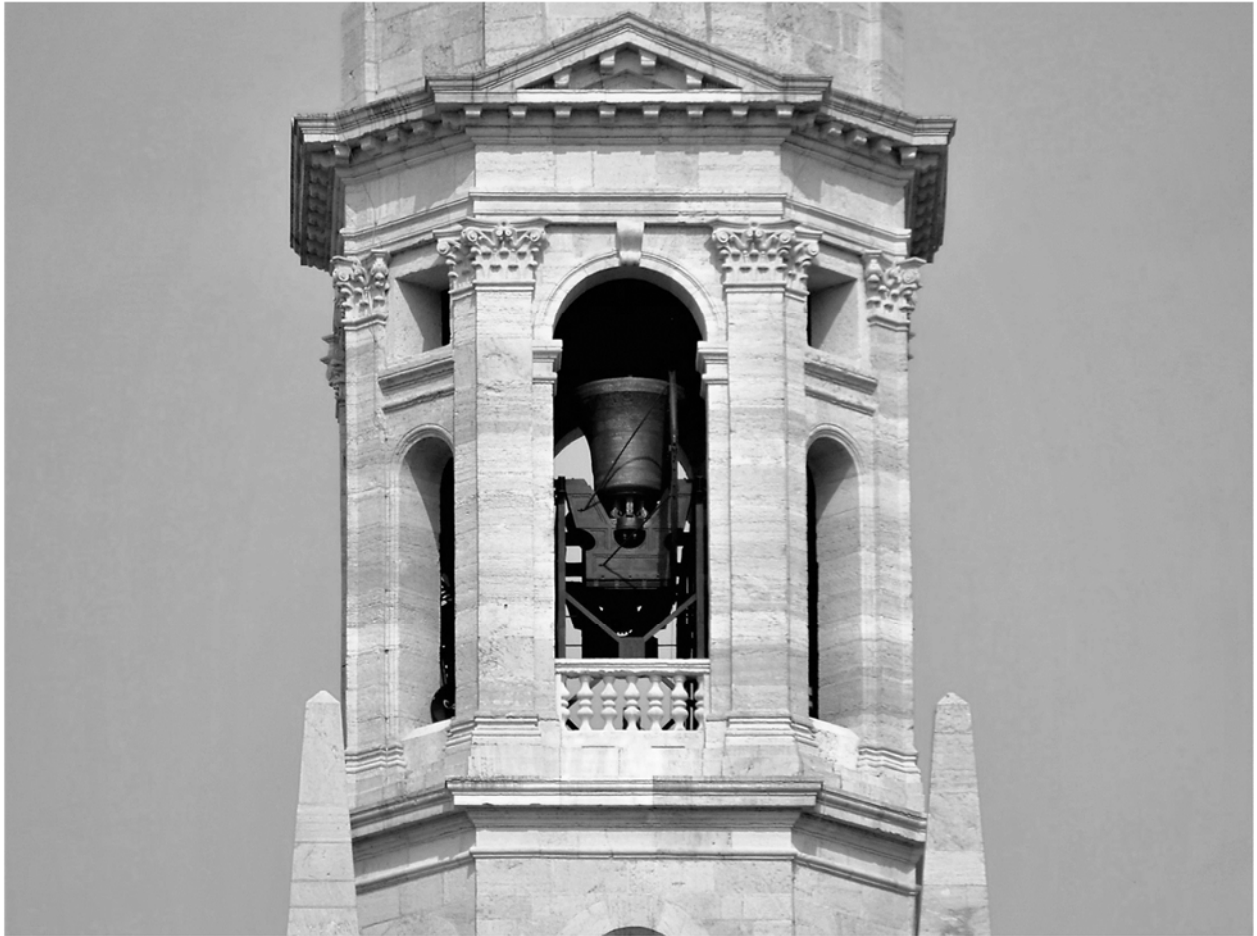
Fig. 7: Bells of Verona Cathedral (Italy) in the “up” position during a manual solemn peal (photo by Matteo Padovani). The main bell, weighing 4566 kg, is the heaviest bell in the world that can be rung by hand in full-circle rotation.
